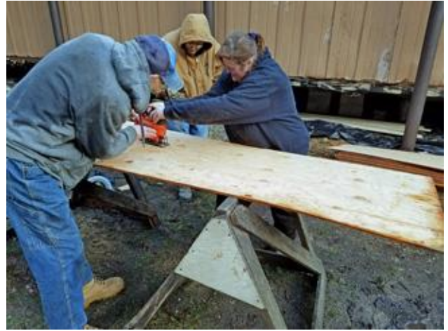
John Boy and Krista guide the jigsaw as it cuts the holes for the vents in the skirting.
