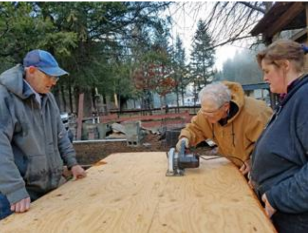
John Boy and Krista hold the plywood for Verne to cut it to fit as skirting around the trailer home.
