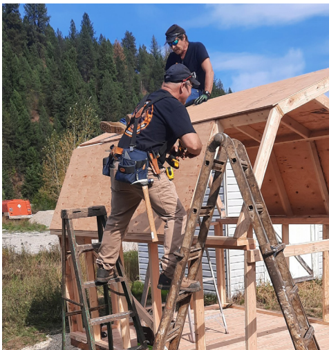
Frank straddles ladders to install sheeting for roof with the help of another volunteer. Volunteers prepare to lift the framed roof onto the walls of the shed.
