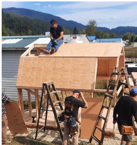
Frank straddles ladders to install sheeting for roof with the help of another volunteer. Volunteers prepare to lift the framed roof onto the walls of the shed.
